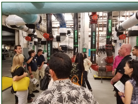
Zack Main leads tour of Waterfront Plaza Chillers.
